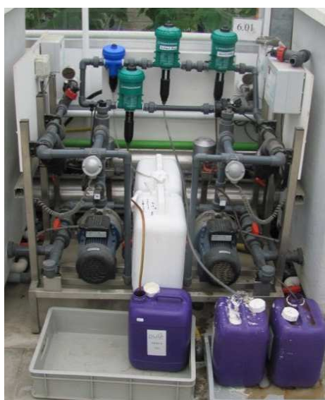
Figure 1. Nutrient dosing of F1, F2 and Endoprotease. Dosatrons in the back.
